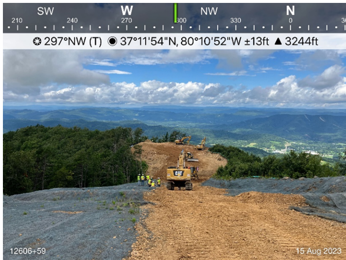
Figure 3: Sta 12606+59, ECD's are in place.
