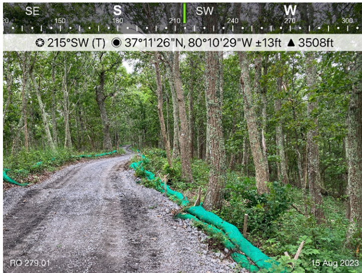
Figure 1: AR RO 279.01, ECD's are in place.
