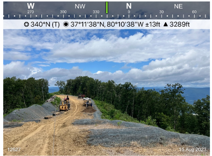
Figure 2: Sta 12627, ECD's are in place.
