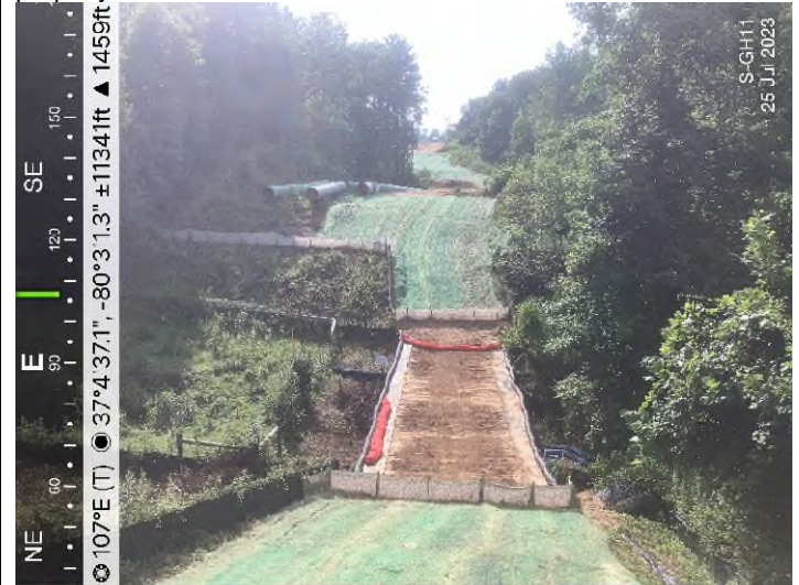
Figure 2: Stream S-GH11 – Controls in place and functioning properly.
