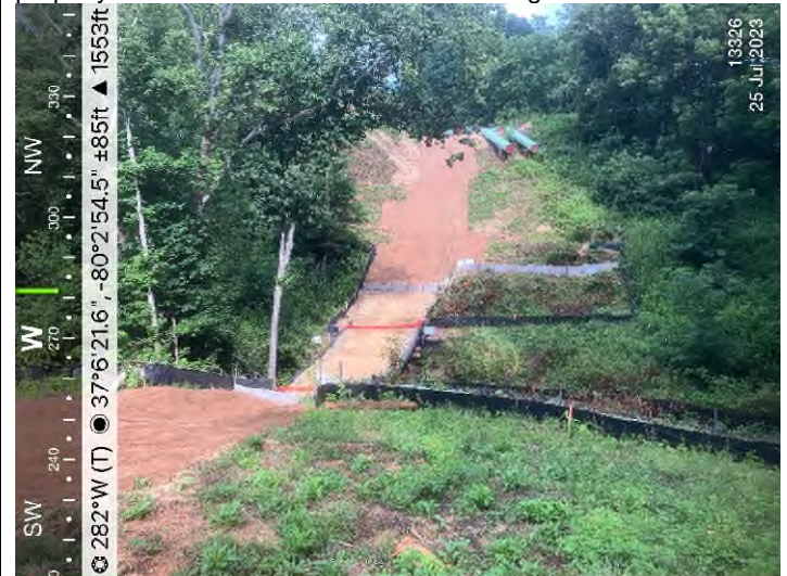
Figure 4: STA 13326+00 – Controls in place and functioning properly. Area stabilized with erosion matting and straw.
