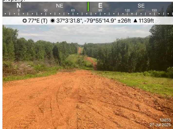
Figure 1: STA 13853+00 – Controls in place and functioning properly.
