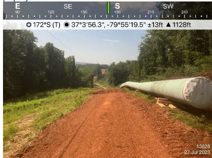
Figure 4: STA 13828+00 – Controls in place and functioning properly.
