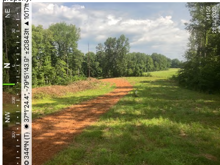
Figure 3: STA 14150+00 – Controls in place and functioning properly.
