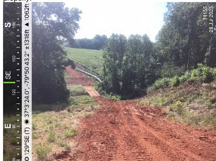
Figure 2: STA 14155+00 – Controls in place and functioning properly.
