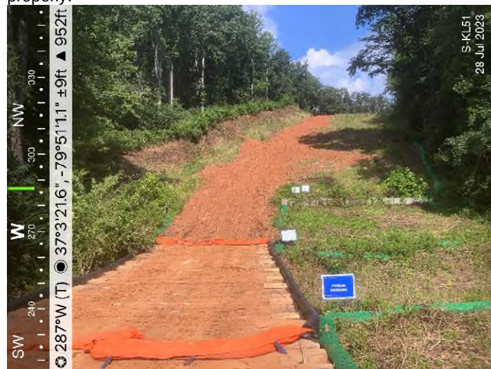
Figure 4: Stream S-KL51 – Controls in place and functioning properly.
