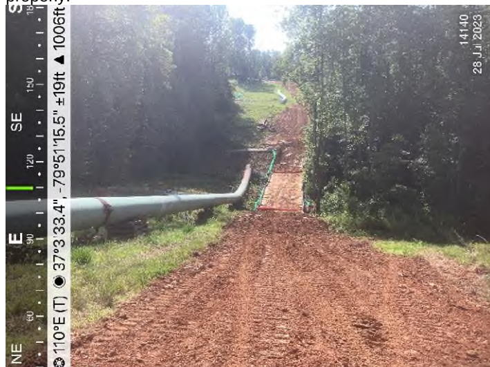
Figure 1: STA 14140+00 – Controls in place and functioning properly.
