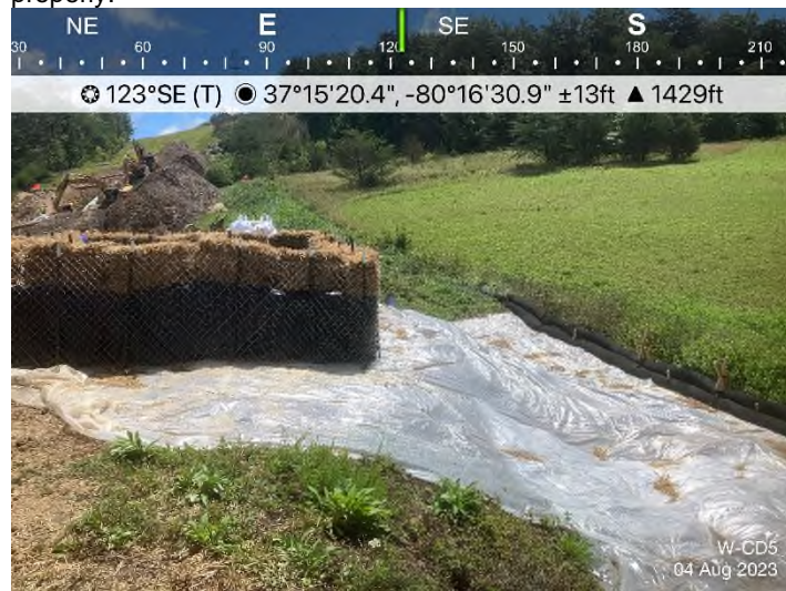
Figure 4: STA 12142+00 – Controls in place and functioning properly.
