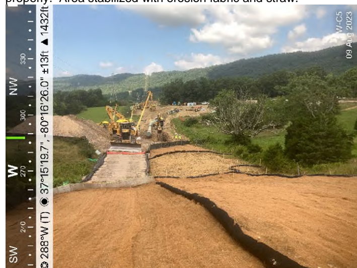
Figure 2: Wetland W-C6 – Controls in place and functioning properly. Area stabilized with erosion fabric and straw.
