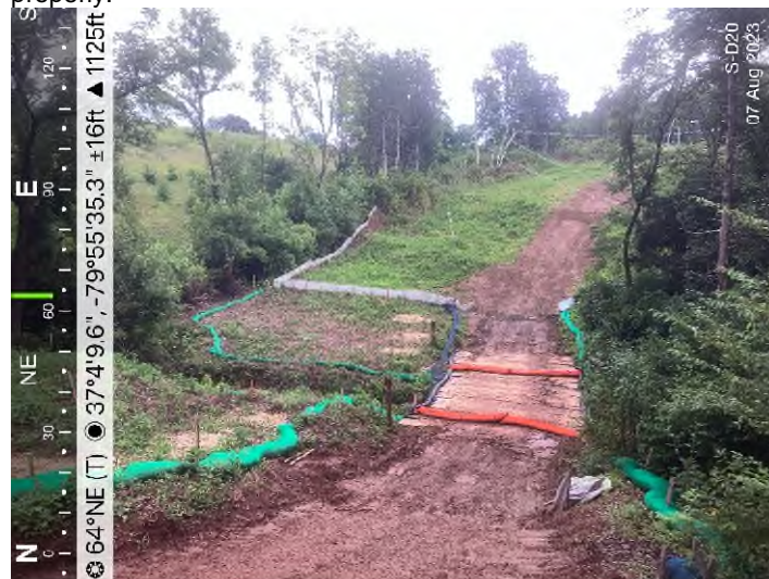
Figure 3: Stream S-D20 – Controls in place and functioning properly.
