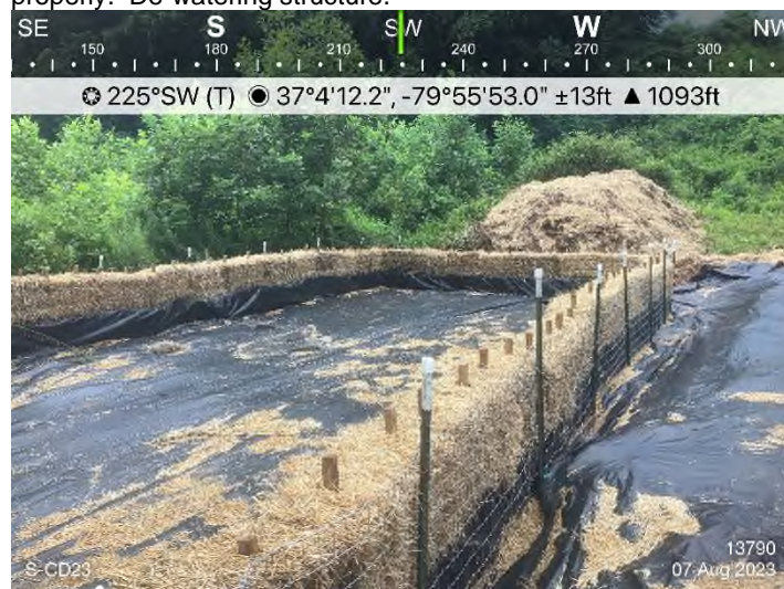
Figure 2: STA 13790+00 – Controls in place and functioning properly. De-watering structure.
