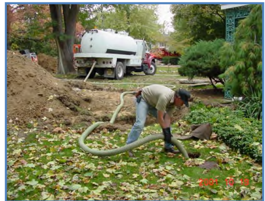
Septic Tank Pump-out
