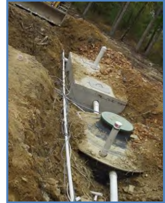
Alternative On-site Sewage Disposal System
