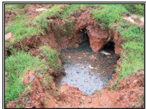
Failed Septic System
