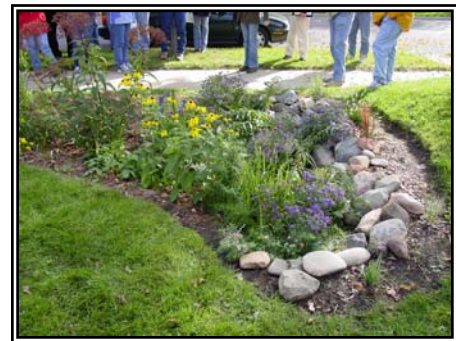
Bioretention (LID Practice)
