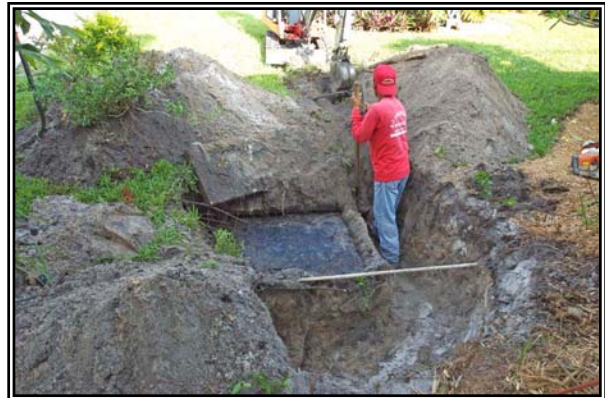
Septic System Repair
