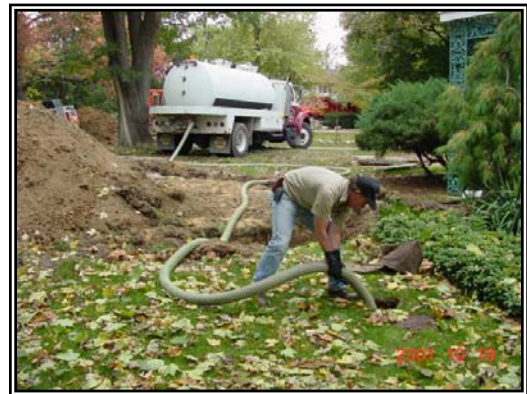
Septic System Pump-out
