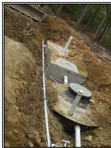
Alternative On-site Sewage Disposal System
