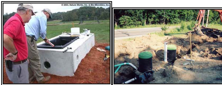
Alternative On-site Sewage Disposal System
