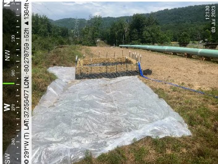
Figure 3: STA 12130+00 – Controls in place and functioning properly.
