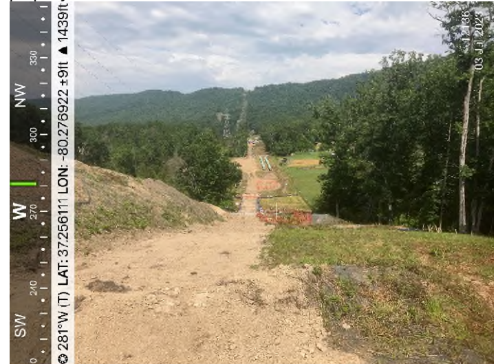
Figure 2: STA 12136+00 – Controls in place and functioning properly.
