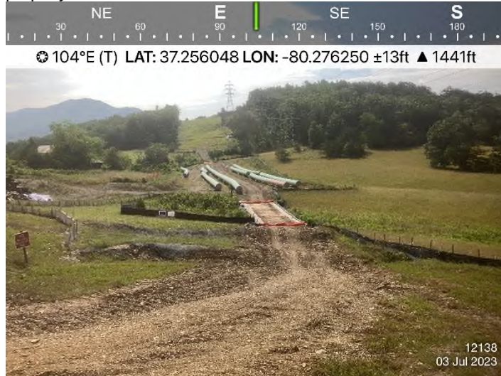
Figure 1: STA 12138+00 – Controls in place and functioning properly.
