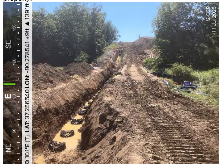
Figure 2: Stream S-C29 – Controls in place and functioning properly.
