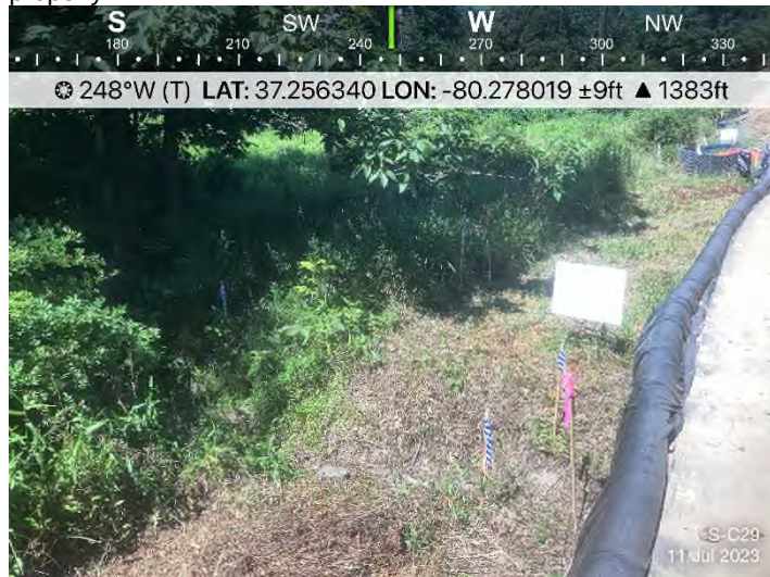
Figure 3: Stream S-C29 - Controls in place and functioning properly.
