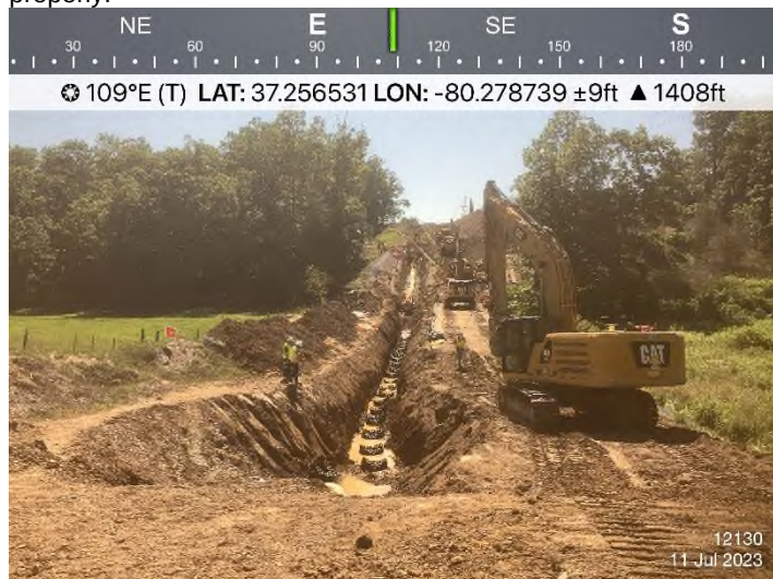
Figure 1: STA 12130+00 – Controls in place and functioning properly.
