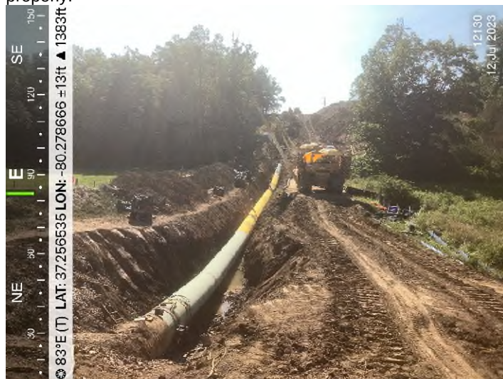
Figure 3: STA 12130+00 - Controls in place and functioning properly.
