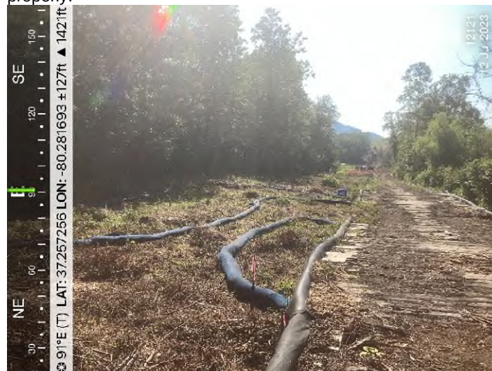
Figure 2: STA 12121+00 - Controls in place and functioning properly.
