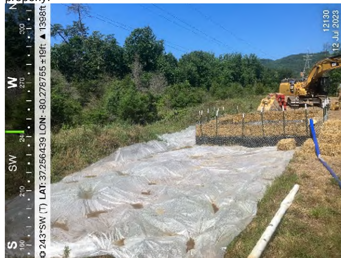
Figure 4: STA 12129+00 - Controls in place and functioning properly.
