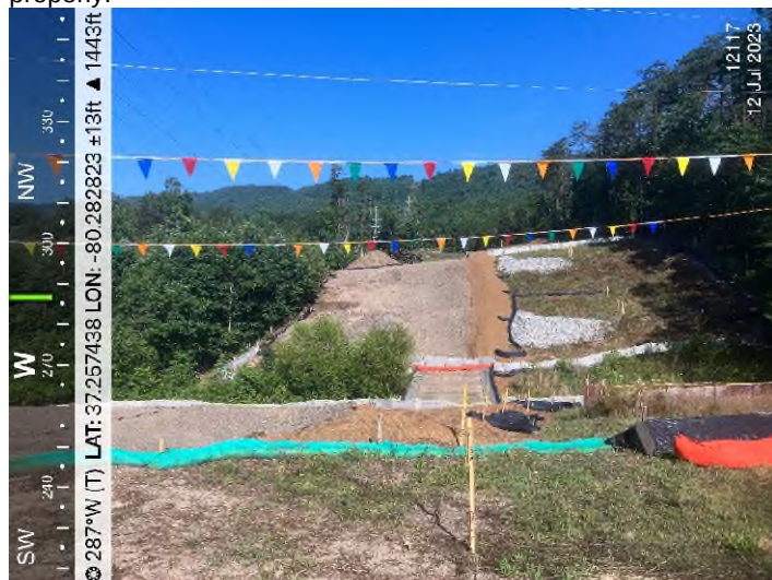
Figure 1: STA 12117+00 – Controls in place and functioning properly.
