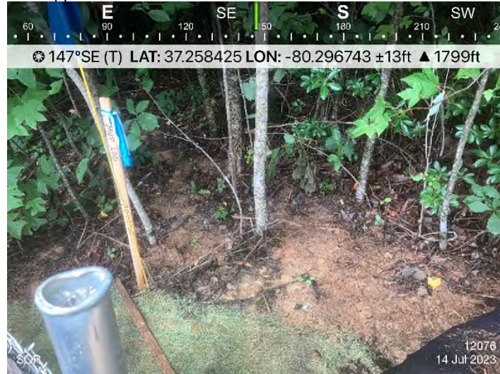
Figure 1: STA 12076+00 – Sediment off ROW. End treatment overtopped.
