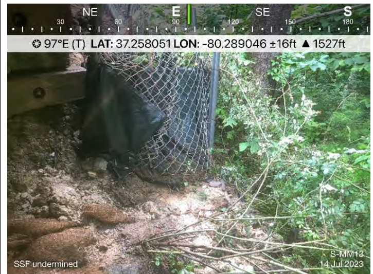
Figure 4: STA 12098+75 – SSF undermined or bypassed.
