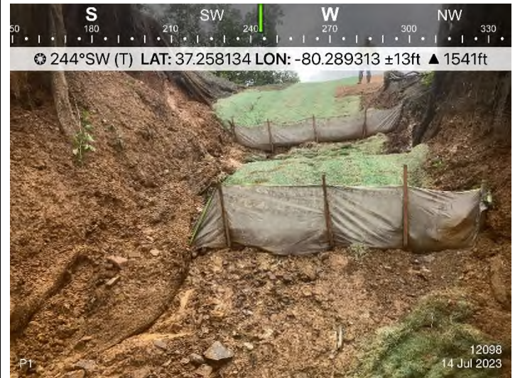
Figure 4: STA 12098+75 – SSF undermined or bypassed.
