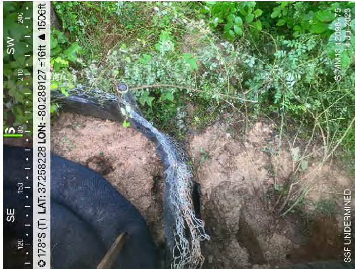
Figure 5: STA 12098+75 – SSF undermined or bypassed.
