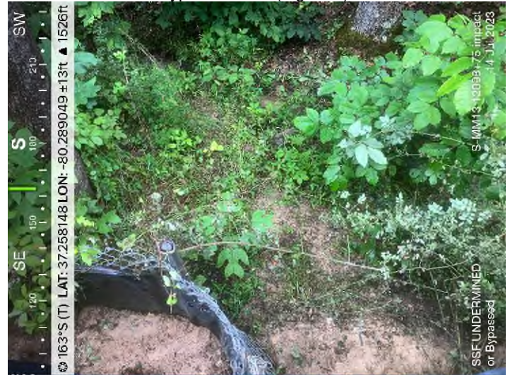
Figure 6: STA 12098+75 – Sediment impacting stream S-MM13 from undermined or bypassed SSF (Figure 5).
