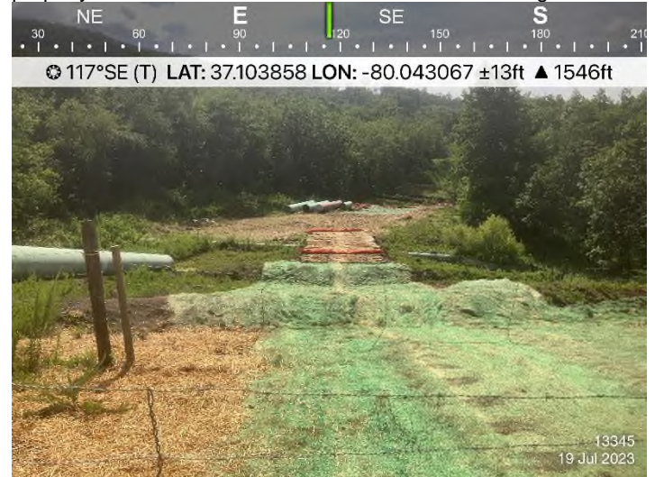
Figure 2: STA 13345+00 – Controls in place and functioning properly. Area stabilized with straw and erosion matting.
