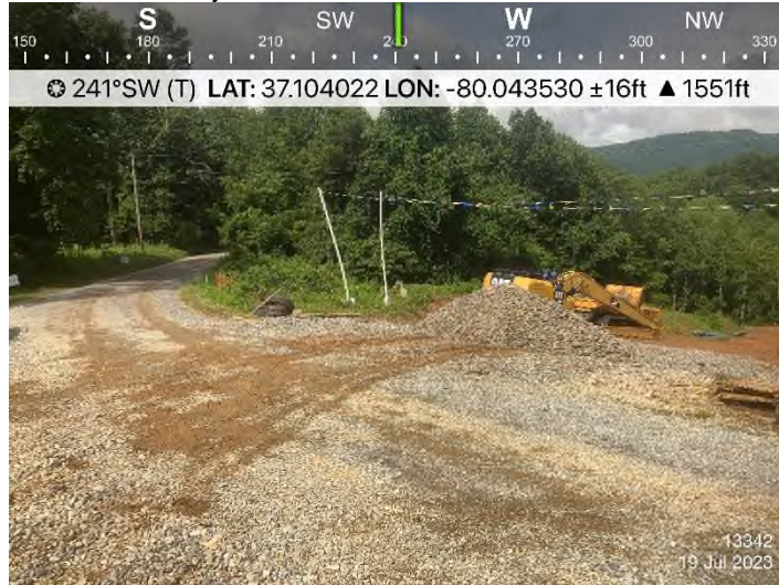
Figure 1: Websters Corner Rd. – Crews adding more stone to RCE and roadway.
