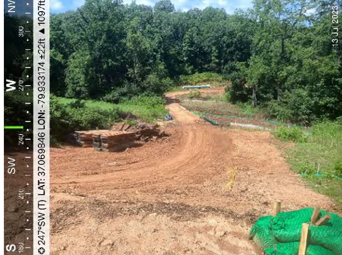
Figure 1: STA 13783+00 – Controls in place and functioning properly.
