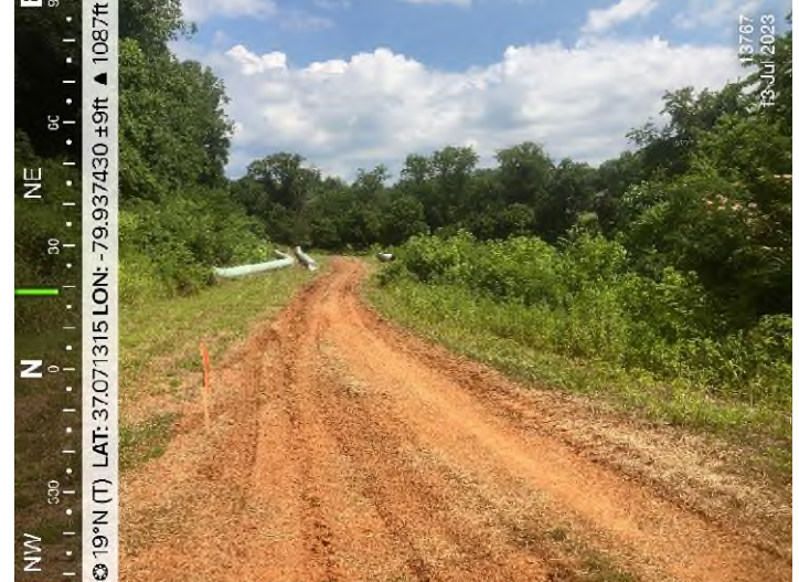
Figure 4: STA 13767+00 – Controls in place and functioning properly.
