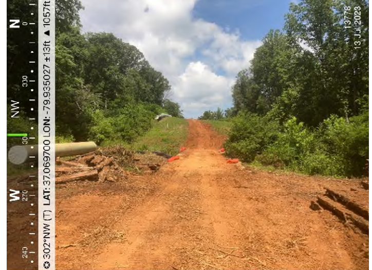
Figure 2: STA 13778+00 – Controls in place and functioning properly.
