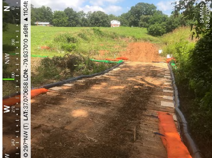
Figure 3: Stream S-MM42 - Controls in place and functioning properly.
