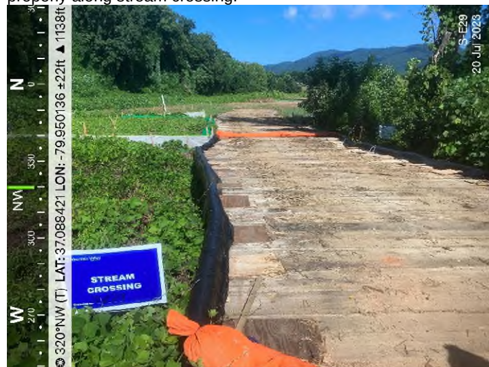
Figure 3: Stream S-E29 – Controls in place and functioning properly along stream crossing.
