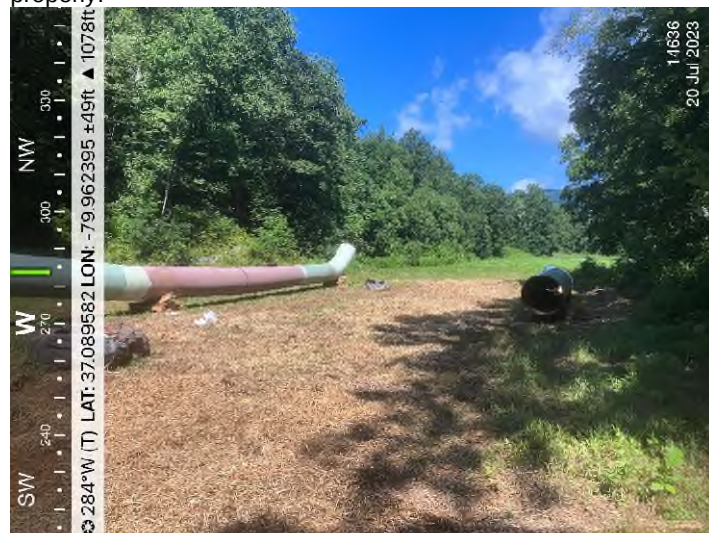
Figure 4: STA 14636+00 – Controls in place and functioning properly.
