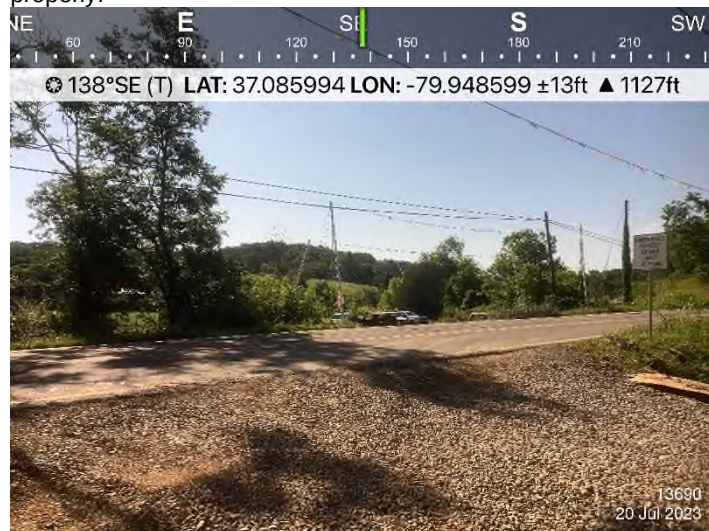
Figure 2: STA 13690+00 – Controls in place and functioning properly.
