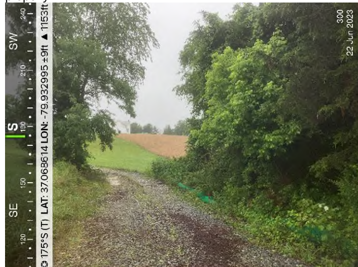
Figure 2: MVP-FR-300 – Controls in place and functioning properly.
