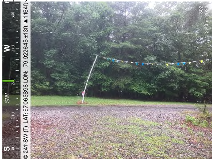
Figure 3: MVP-FR-302 – Controls in place and functioning properly.
