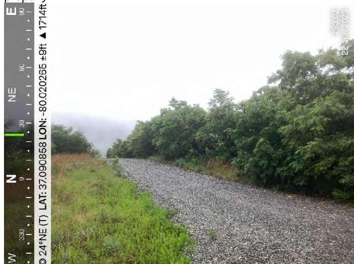
Figure 1: MVP-FR-293.02 – Controls in place and functioning properly.
