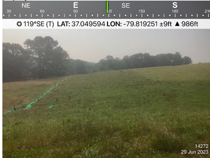
Figure 1: STA 14272+00 – Controls in place and functioning properly.
