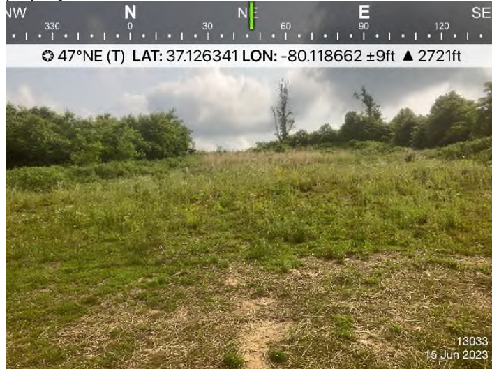
Figure 1: STA 13033+00 – Controls in place and functioning properly.
