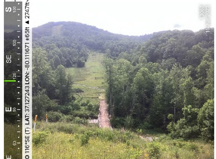
Figure 4: STA 13060+00 – Controls in place and functioning properly.
