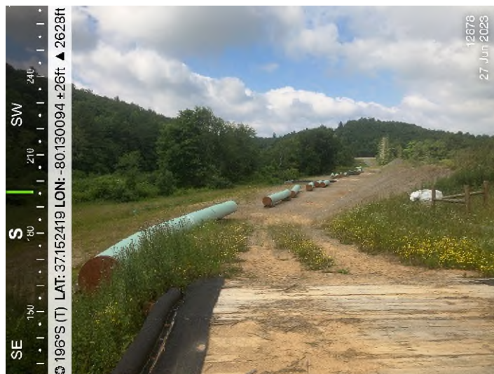
Figure 3: STA 12878+00 – Controls in place and functioning properly. Area stabilized with straw and blanket matting.
