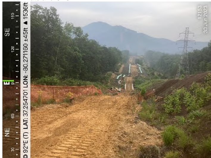
Figure 1: STA 12153+00 – Crews clearing brush, installing new timber mats and CFS.
