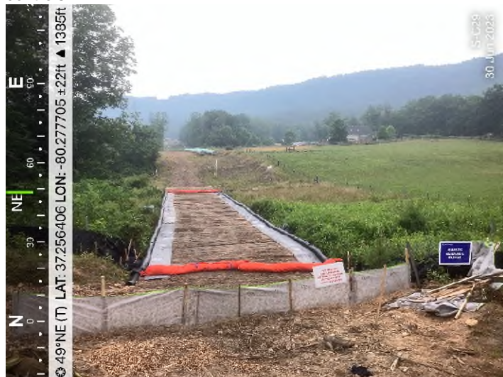
Figure 3: Stream S-C29 – Controls in place and functioning properly. Recently replaced timber mat crossing and perimeter controls.
