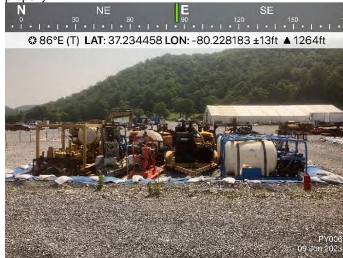
Figure 4: Pipeyard 006 – Controls in place and functioning properly.
