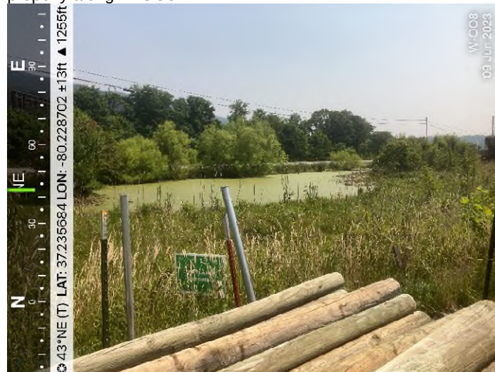
Figure 2: Pipeyard 006 – Controls in place and functioning properly along W-008.
