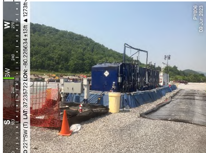
Figure 1: Pipeyard 006 – Controls in place and functioning properly.
