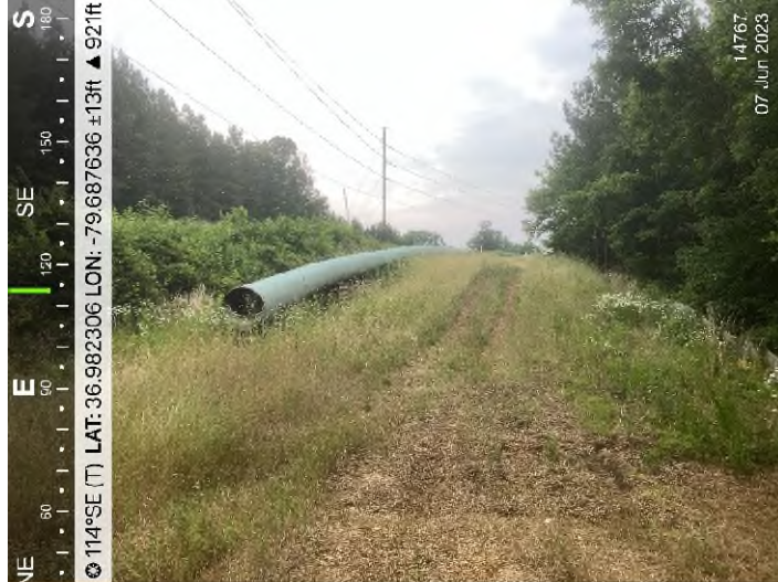
Figure 1: STA 14767+00 – Controls in place and functioning properly.
