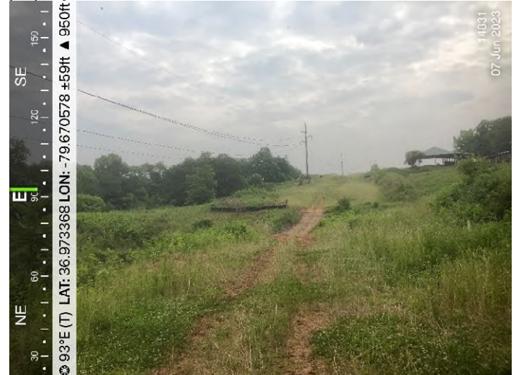
Figure 4: STA 14831+00 – Controls in place and functioning properly.
