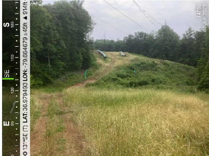
Figure 3: STA 14780+00 – Controls in place and functioning properly.
