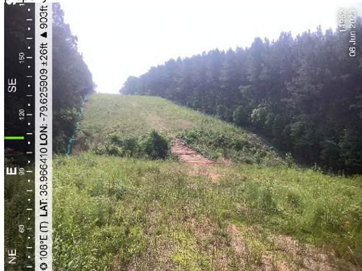
Figure 3: STA 14962+00 – Controls in place and functioning properly.
