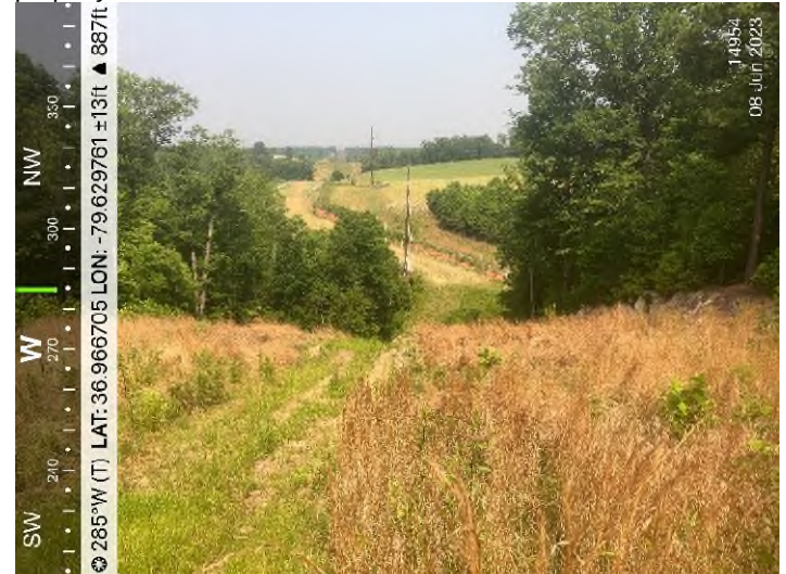
Figure 2: STA 14954+00 – Controls in place and functioning properly.
