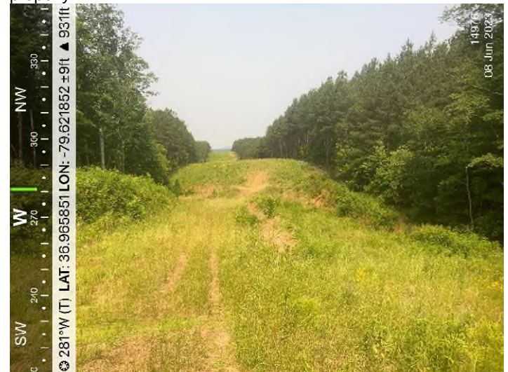
Figure 4: STA 14978+00 – Controls in place and functioning properly.
