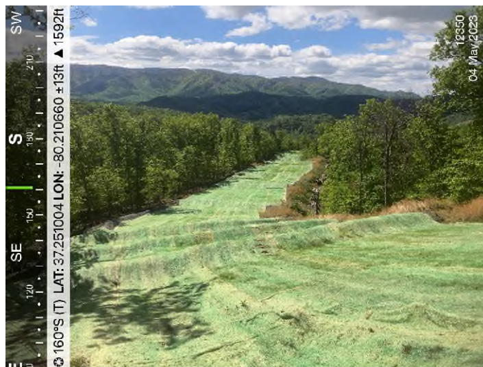
Figure 3: STA 12350+00 – Controls in place and functioning properly.
