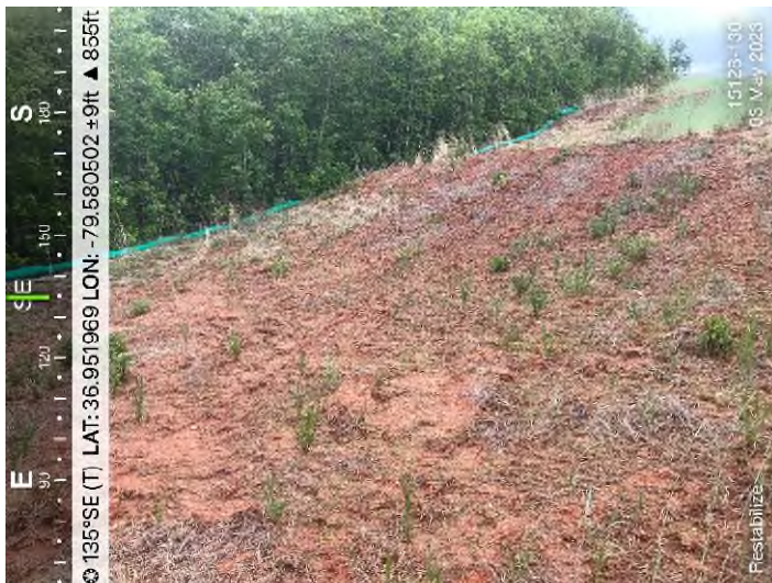
Figure 3: STA 15128+00 to 15130+00 – Re-stabilization needed.
