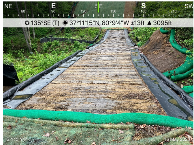
Figure 4: Designated crossing S-Y13 & S-Y14, ECD's are in place.
