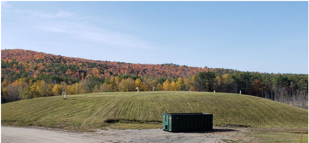
Figure 1:1 Covered Landfill with Gas Ventilation Pipes
