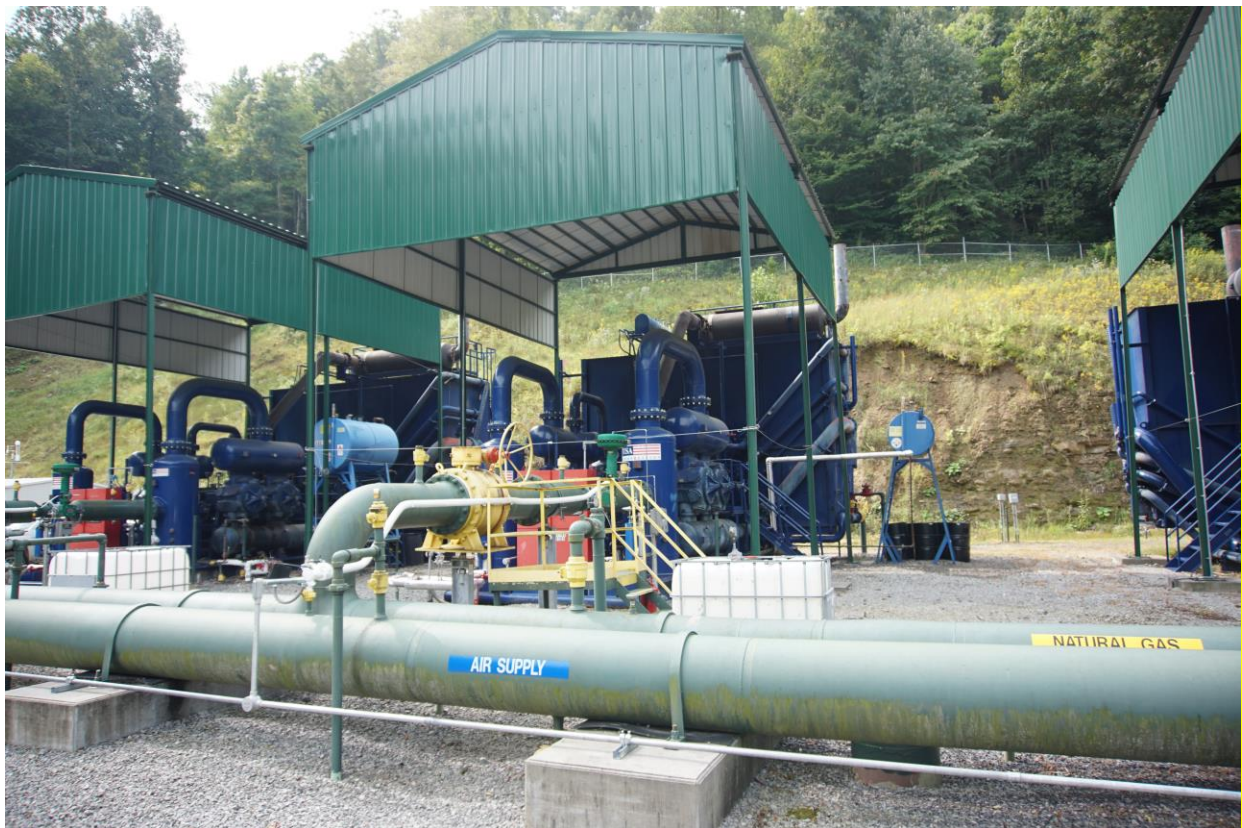
Figure 1:4 CAT3516 Tale Unit at Compressor Site
