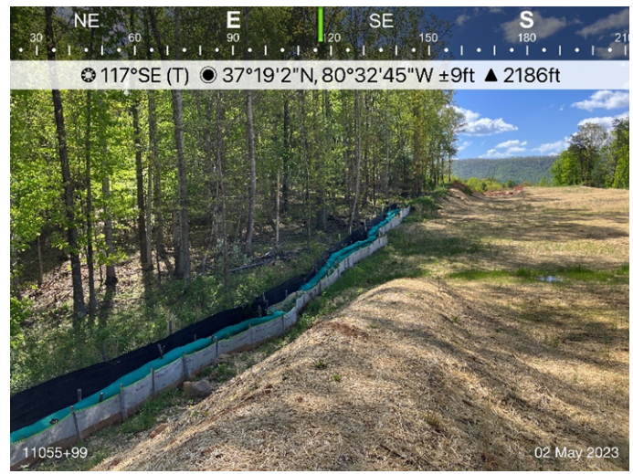
Figure 4: St11055+99 ECD's are in place.
