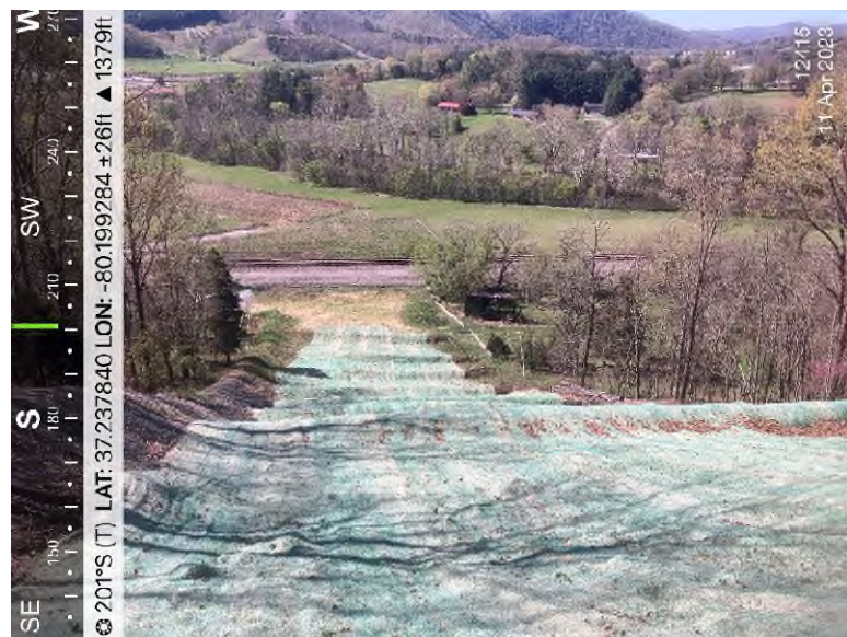
Figure 4: STA 12385+00 – Controls in place and functioning properly.
