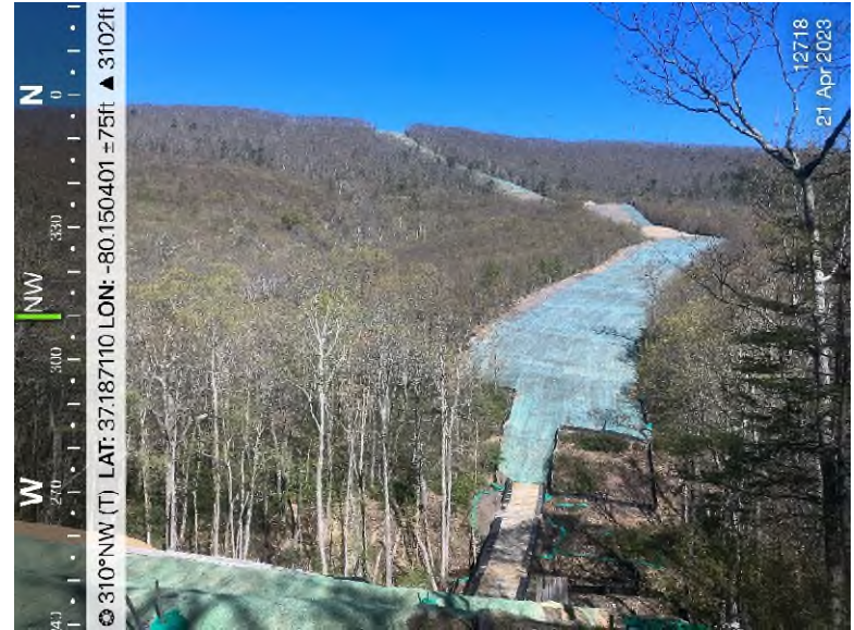
Figure 4: STA 12706+00 to 12707+00 – Restabilization needed.
