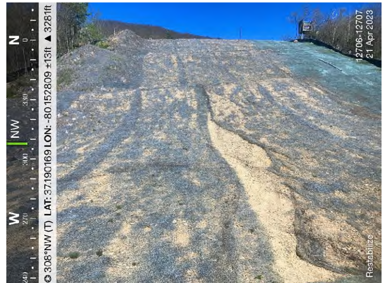
Figure 4: STA 12706+00 to 12707+00 – Restabilization needed.
