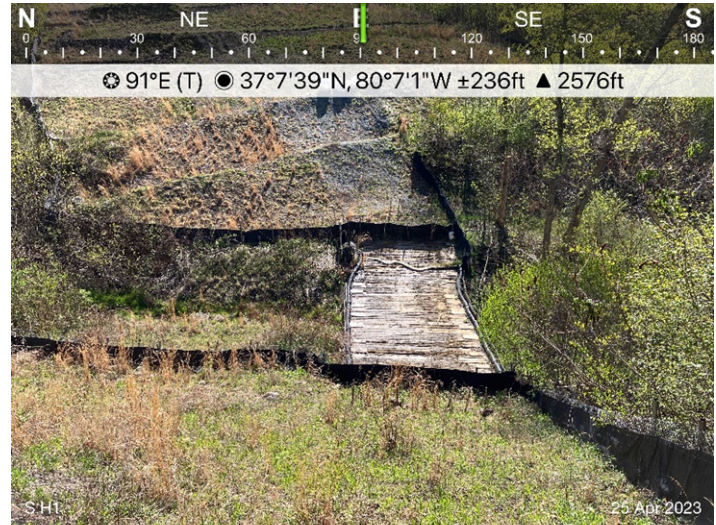
■ Figure 2: Designated crossings S-H1, ESC measures in place.
