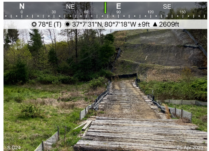
■ Figure 4: Designated crossing S-G24, ESC measures in place.
