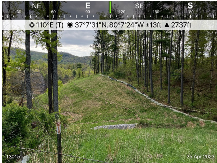
■ Figure 1: Sta 13015, ECD's are in place and functioning.
