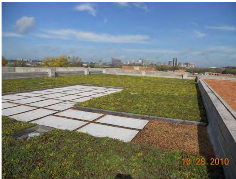
Figure 5.2 Vegetated Roof installed on the Richmond Wastewater Treatment Plant in Richmond, VA.
