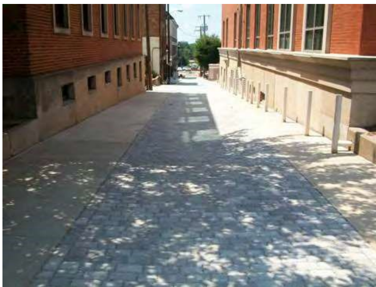
Figure 5.1 Pervious pavement installed in the 5 th Street Alley in Richmond, VA.
