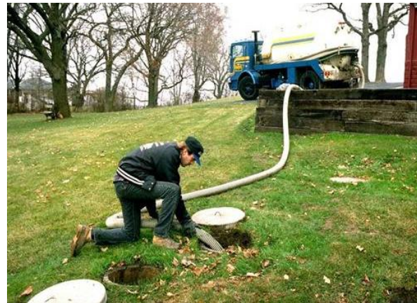
Septic tank pumpout.
