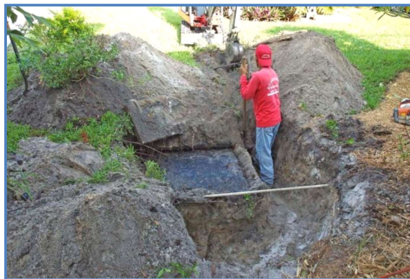
Septic System Repair
