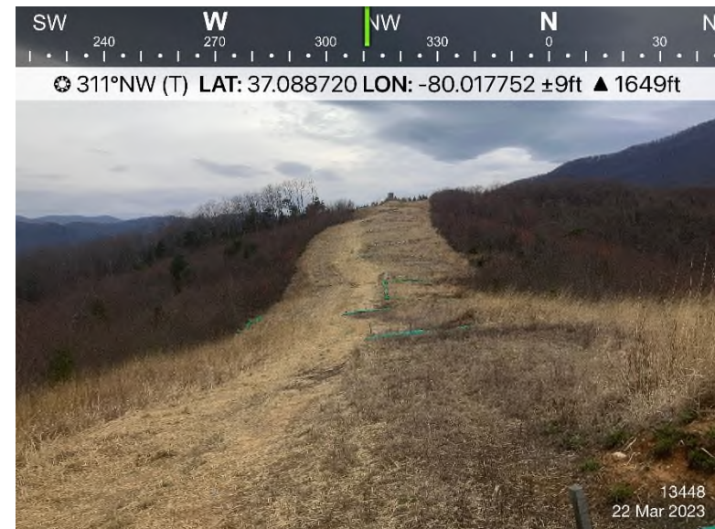
Figure 3: STA 13448+00 – Controls in place and functioning properly.
