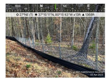
Figure 2: Designated crossings S-C33, S-C36 &W-C11, ESC measures in place.
