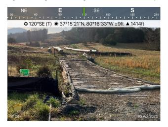
Figure 4: Designated crossing S-C25, ESC measures in place.
