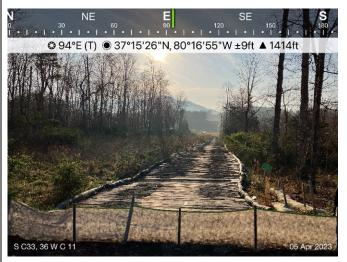
Figure 3: Designated crossing W-C6, ESC measures in place.
