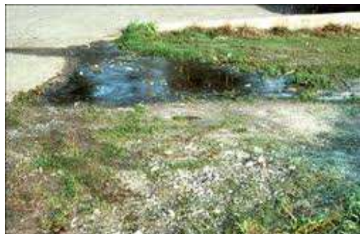
Figure 5. Failing septic system
