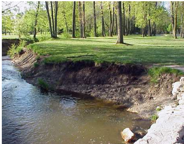
Figure 13. An eroding streambank
