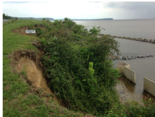
Beach erosion structures.
