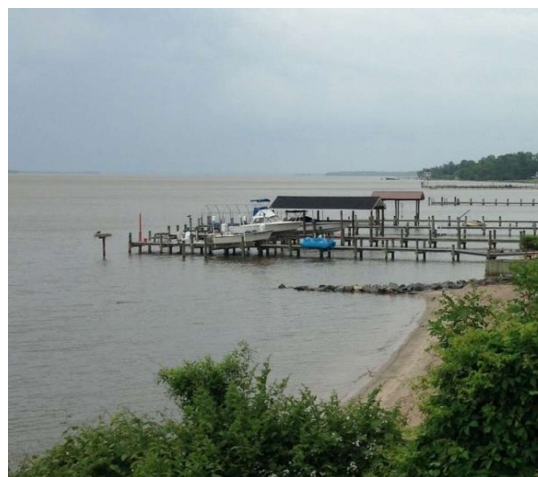
Piers near 6th Street.
