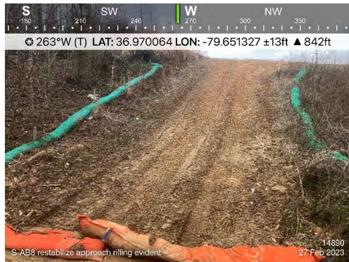
Figure 3: STA 14890+00 – Re-stabilize travel lane CIS S-AB8.
