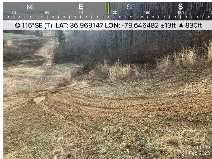
Figure 4: STA 14905+00 to 14907+00 – Re-stabilize travel lane.
