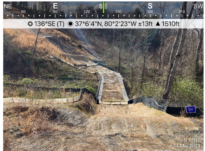
Figure 2: Designated crossing S-RR11, ESC in place.
