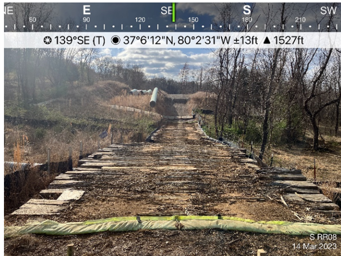
Figure 1: Designated crossing S-RR08, ESC in place.
