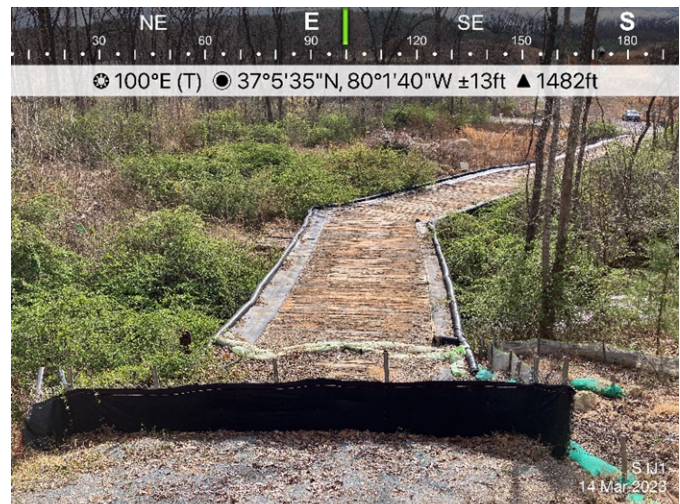
Figure 4: Designated crossing S-IJ1, ESC in place.
