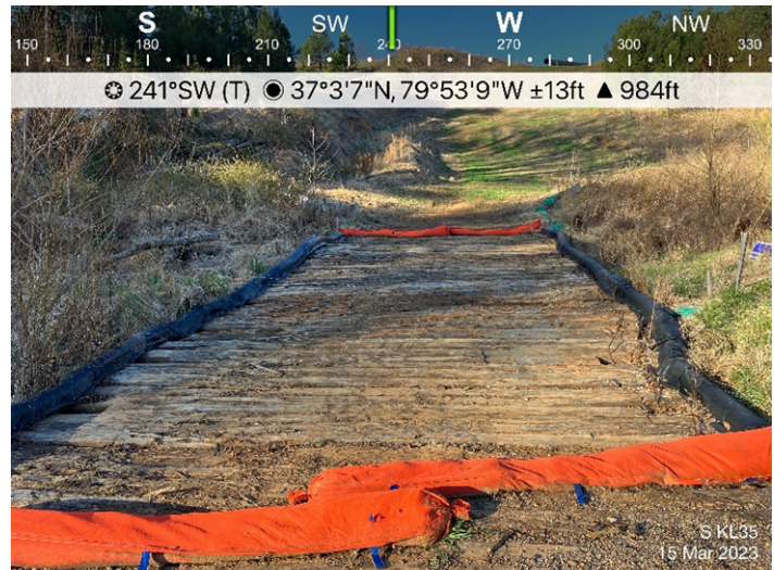
Figure 4: Designated crossing S-KL35, ESC in place.
