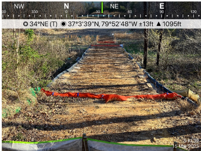
Figure 3: Designated crossing S-KL39, ESC in place.
