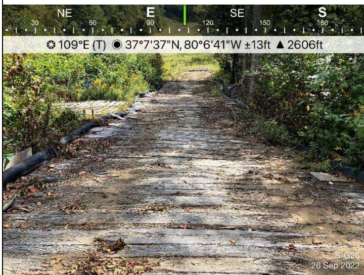
Figure 3: Designated crossing S-G26, ECD's are in place.
