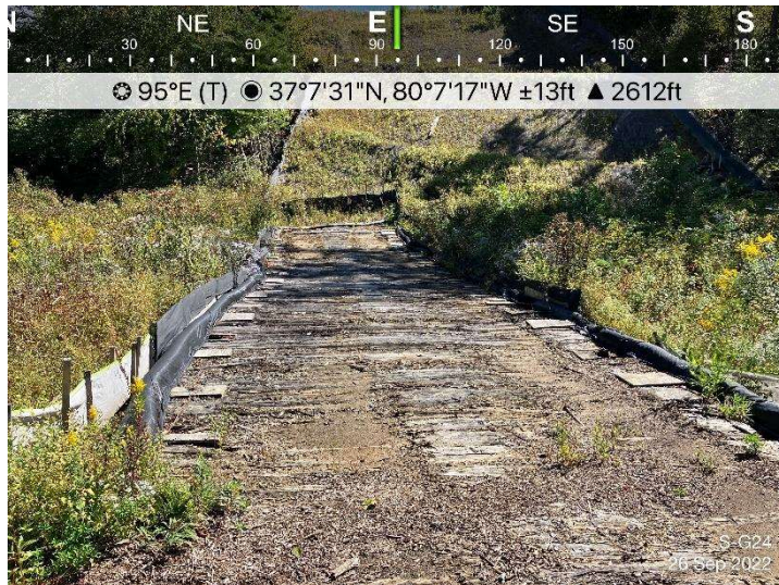
Figure 1: Designated crossing S-G24, ECD's are in place.
