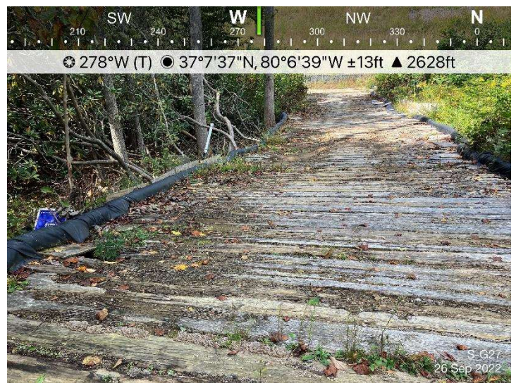
Figure 4: Designated crossing S-G27, ECD's are in place.
