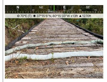
Figure 2: Designated crossing W-C6, ECD's are in place.
