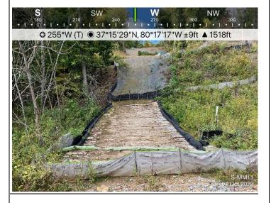
Figure 4: St 12170, ECD's are in place and functioning.
