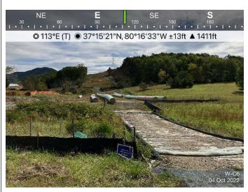
Figure 3: Designated crossing S-MM11, ECD's are in place.
