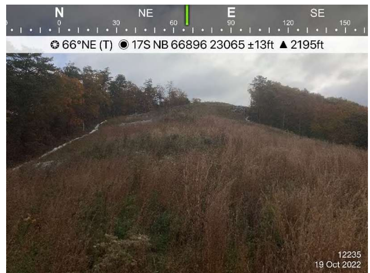
Figure 4: STA 12235+00 – Permanent vegetation is mature, uniform and will inhibit erosion.
