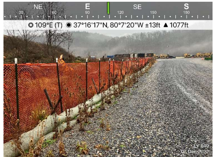
Figure 4: ECD remains in place and functioning at LY049.
