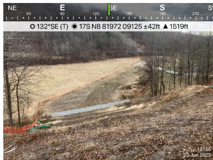
Figure 4: STA 13188+00 – Controls in place and functioning properly.
