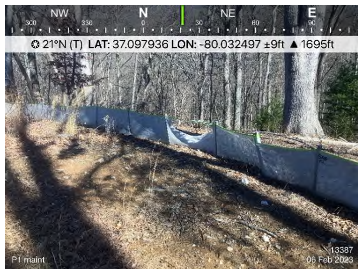
Figure 3: STA 13370+00 – P1 maintenance needed.
