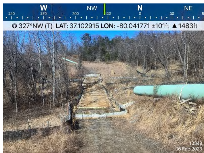
Figure 4: STA 13349+00 – Controls in place and functioning properly.
