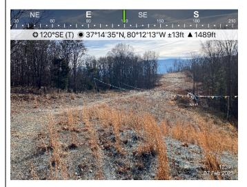
Figure 2: Designated crossing S-0016, ECD's are in place and functioning.
