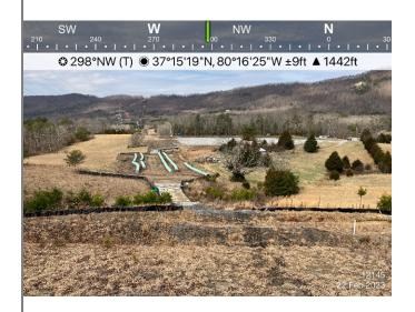
Figure 2: Designated crossing W-C5, ECD's are in place and functioning.
